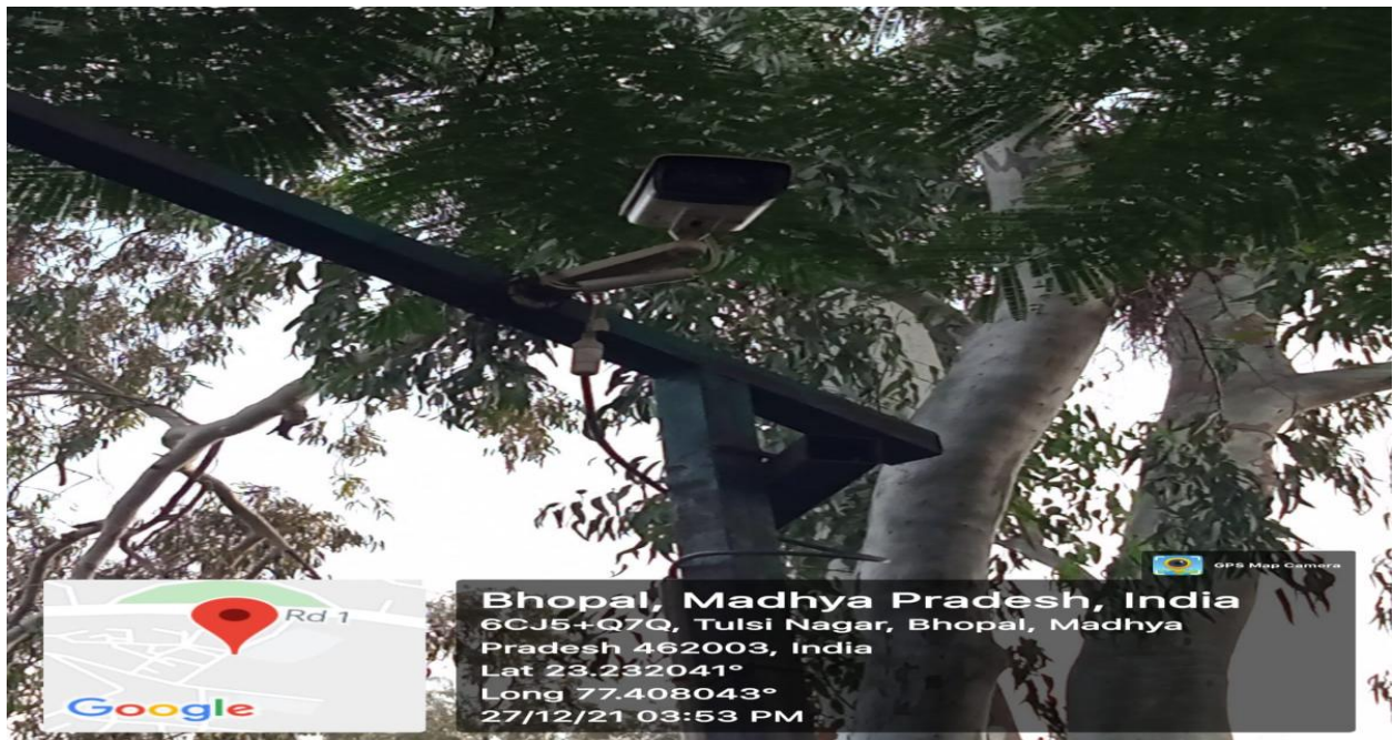
CCTV at Entrance
